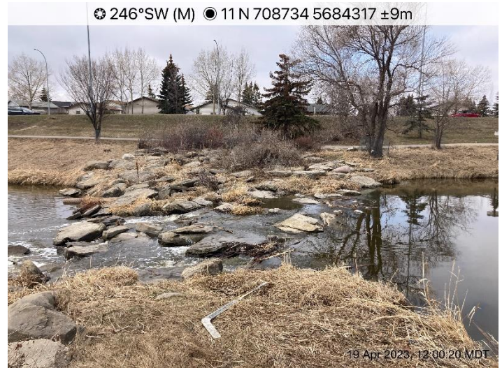
Figure 6-3. Overview photos of the rock weir structures within the Waterstone-Summerhill Area that have created deepwater pools within Nose Creek.
