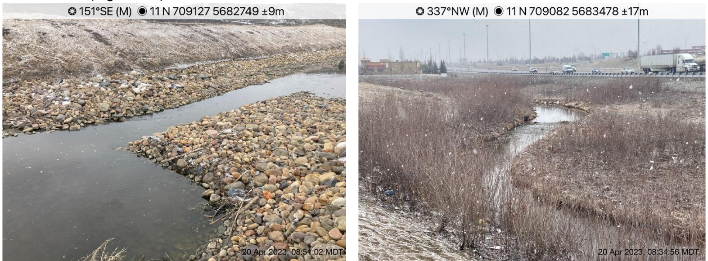
Figure 7-7. Representative examples of a constructed channel restriction (left) and pool-riffle transitions which may act as an anchor point for future beaver dams.
