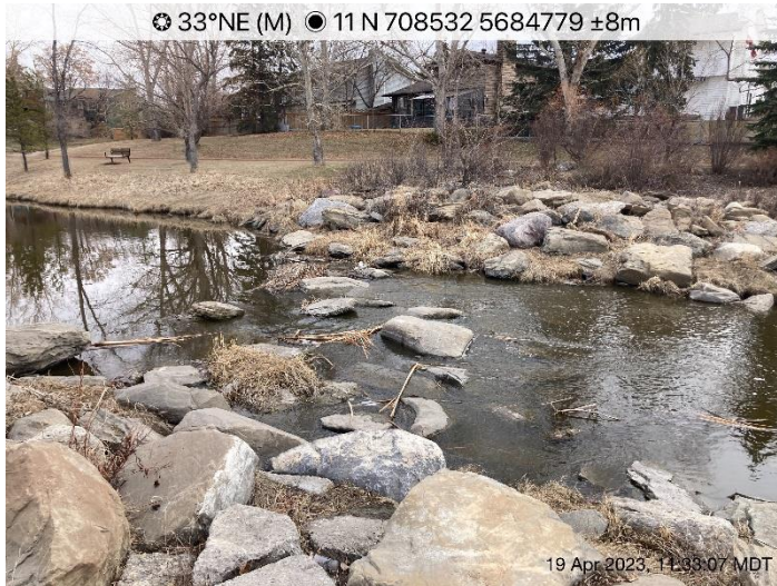
Figure 6-3. Overview photos of the rock weir structures within the Waterstone-Summerhill Area that have created deepwater pools within Nose Creek.
