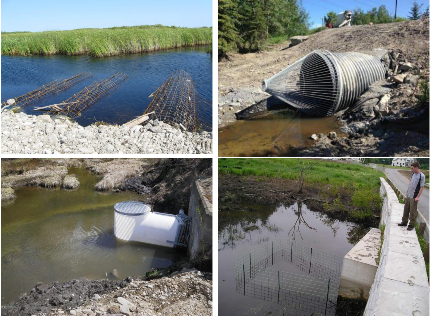
Figure 4-2. Examples of commercially available culvert protection, Beaver Stop (top-left, photo: armtec.com), Beavercone (top-right, photo: beavercone.com), beaverproof add-on (bottom-left, photo: beaverproofaddon.com) and trapezoidal culvert fencing (bottom-right, photo: beaversolution.com)
