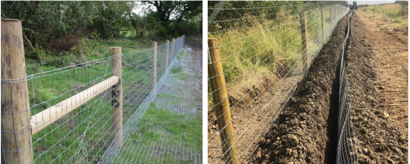
Figure 4-1. Example of exclusion fencing with skirting to discourage digging (left, from Campbell-Palmer et al., 2013) and trenched fencing, prior to backfilling and installation of fence skirting (right, from https://www.sanctusltd.co.uk/ )
