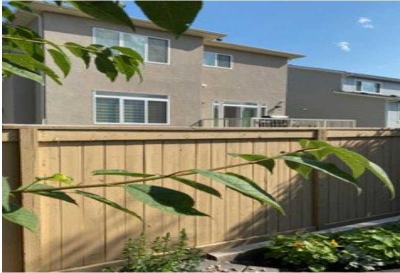
Photo 2 - back yard privacy issues cont'd
