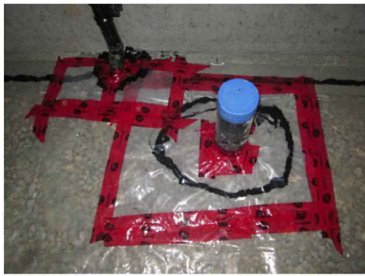
EXAMPLE OF SEALED PENETRATIONS POLY SEALED AROUND PIPES, PIPES SEALED AT SLAB SURFACE.
