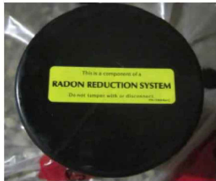
EXAMPLE OF CAP LABEL PIPE NOT TO BE USED FOR ANY OTHER PURPOSE.
