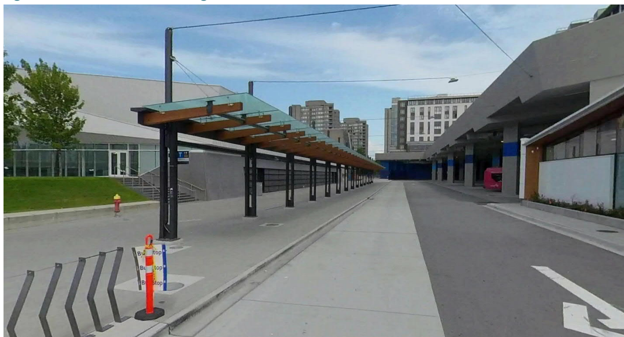
Figure 18: TransLink UBC Exchange Linear Platform
